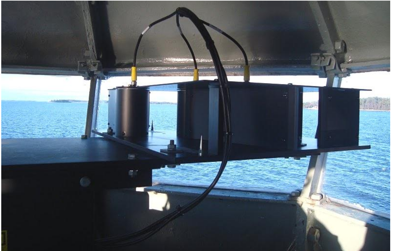
Picture 5. Sector Lantern E8264.RWG.LC-F3138 installed inside a lantern room at Heponiemi, Finland. The picture shows one half of the lantern. Sighting pins are visible in picture centre.
